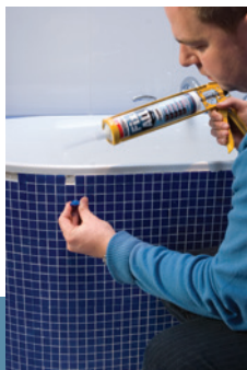
WORKS ON WET AREAS
