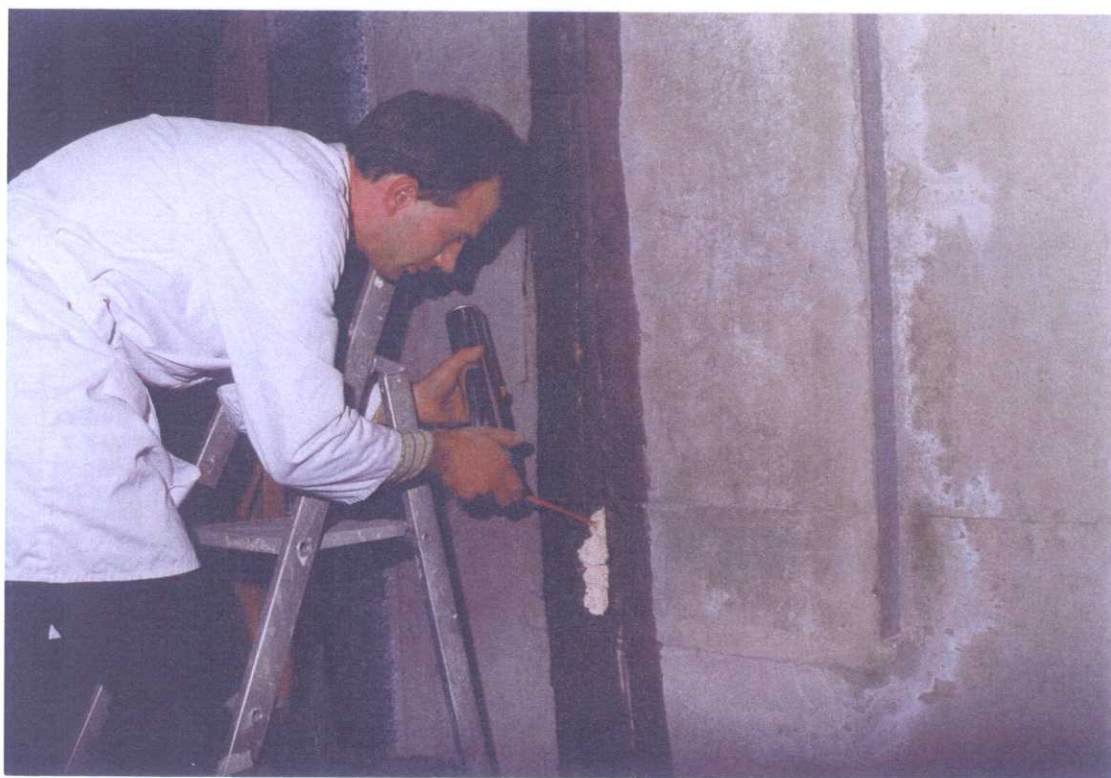
Photo of the face exposed to fire after elimination of the surplus and bringing the seals flush
